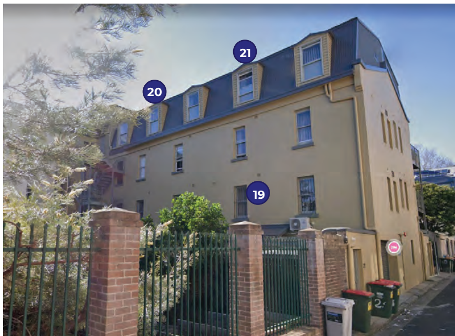
Figure 19 Viewpoint locations from apartments at 21-23 Challis Avenue
